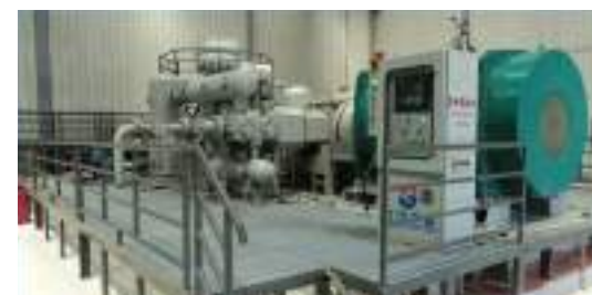
Natural Gas Storage
